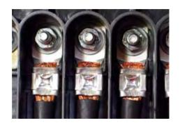
The figure shows an adequate ring-type lug on the left side and an unsuitable standard lug on the right side.
